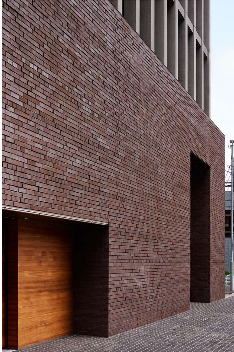
heavily textured bricks custom-made in Hekinan, Aichi Prefecture, compose the south facade
